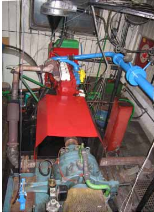
Fig.1 Non-conventional cooling circuit of the engine
